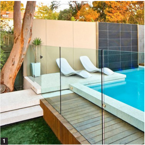
Glass pool fence to perimeter of rooftop
