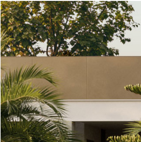
Steel panel fence to conceal services
