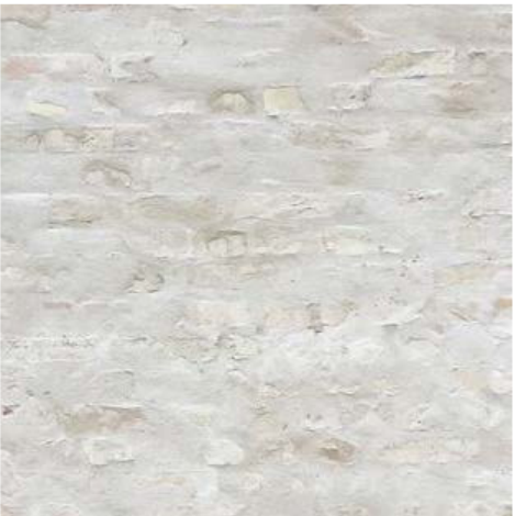
Bagged brick to built in seating wall
